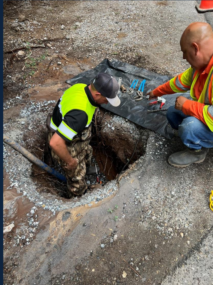
Top Left: Spruce service line break excavation by Curtis Smith and Rick Diaz.
